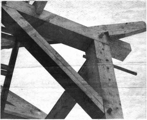
The upper corner of the Whitneyville Library's new cupola shows the old time craftsmanship which is going into the duplicate. Mortise and Tenon joinery of large beams made todays  $2 \times 4$ 's look like toothpicks. Notice the pegging of the joints rather than using nails. (Dirsa Photo)
