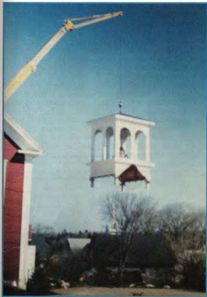
Replacing the restored Cupola to the Whitneyville School roof in Whitneyville, Maine.
