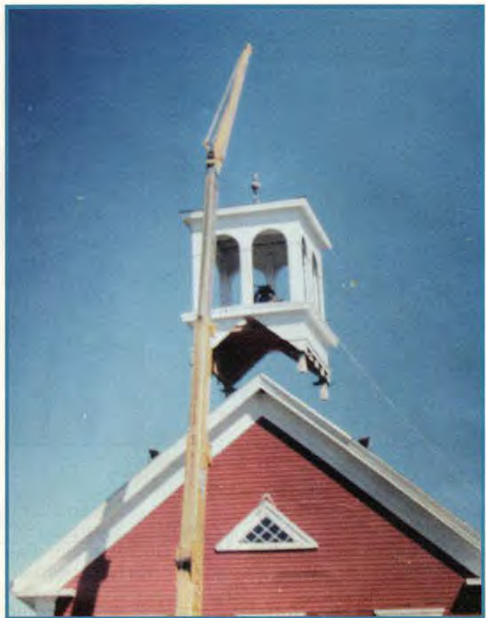
Replacing the restored Cupola to the Whitneyville School roof in Whitneyville, Maine.
